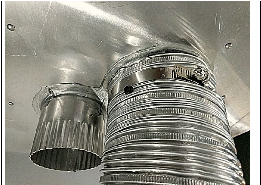
Vent Cap Flex Connection Hose Clamp first. Secure w/ Screw above Hose Clamp
