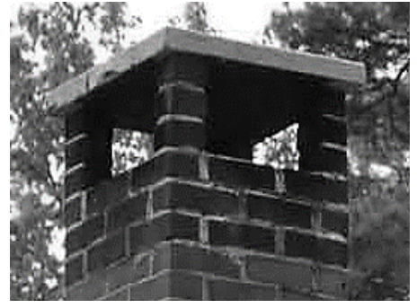
Concrete Cap Chimney Top
